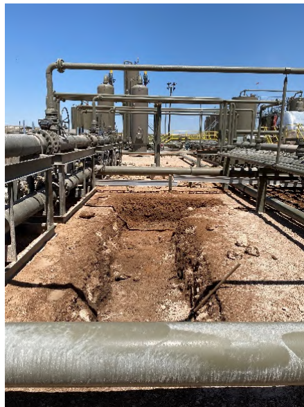
Photograph 4: View east of hydro vacuum excavation
