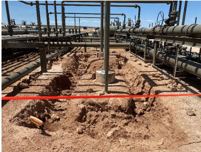
Photograph 3: View west of hydro vacuum excavation, red line in forefront is reflective tape.
