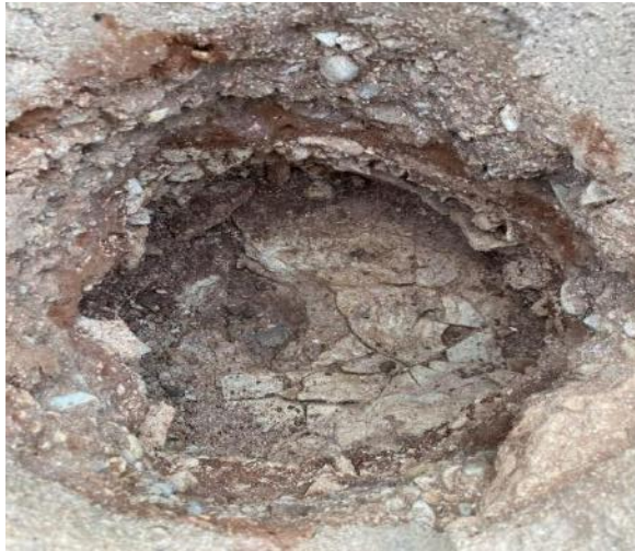
Photograph 4: View of formation material within the lined steel berm.
