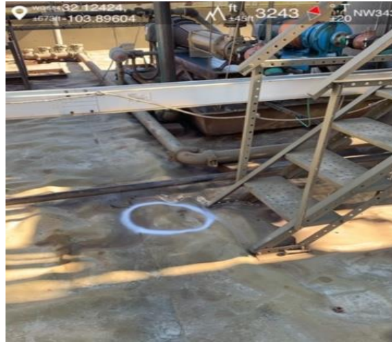
Photograph 1: View of the breached area within the subject release area following recovery of produced water within containment.
