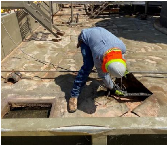
Photograph 5: Injecting Microblaze beneath liner incision prior to repair.
