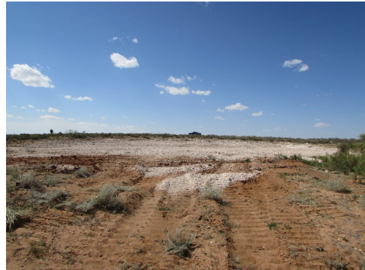
Backfilled and seeded road area 07/10/14
