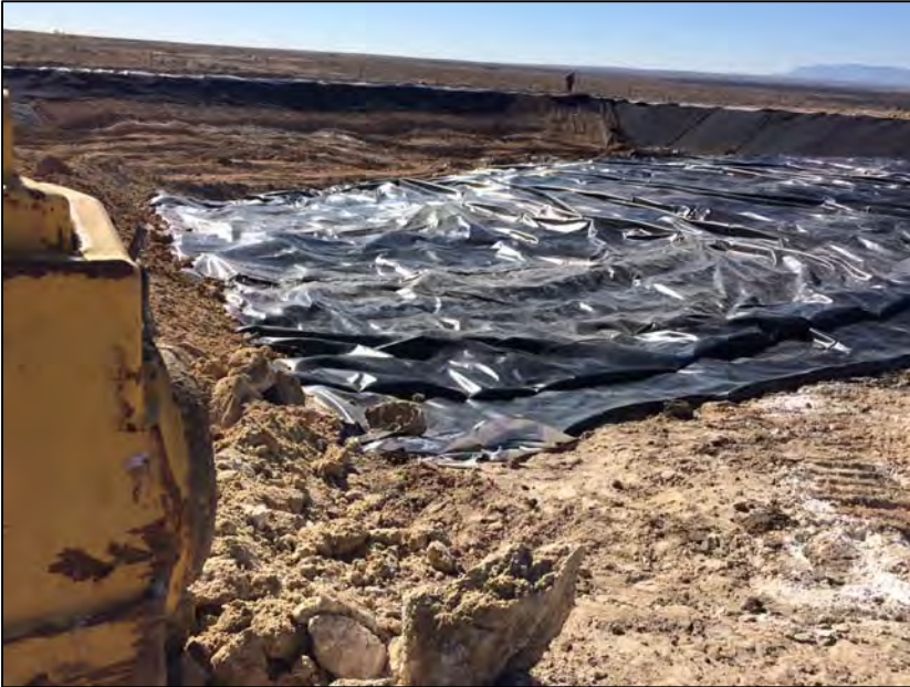
Installing liner over cuttings and backfilling 12/13/2017
