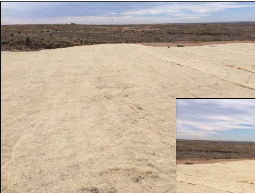
Erosion control blanket over backfilled surface 3/9/2018
