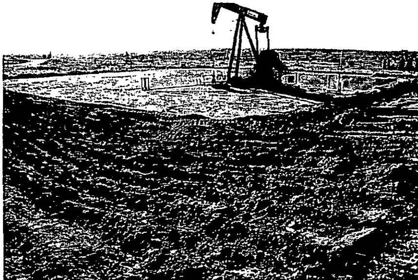
Corners rounded off to gain more in reclamation since these areas are not used for daily operations. IR followed plan in AAPD with IR added to the south side taking to a 3:1 slope. Pad is bermed.
