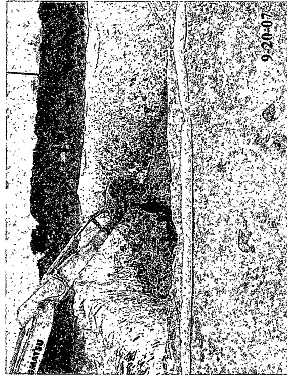
Solidified mud being placed in the burial pit.
