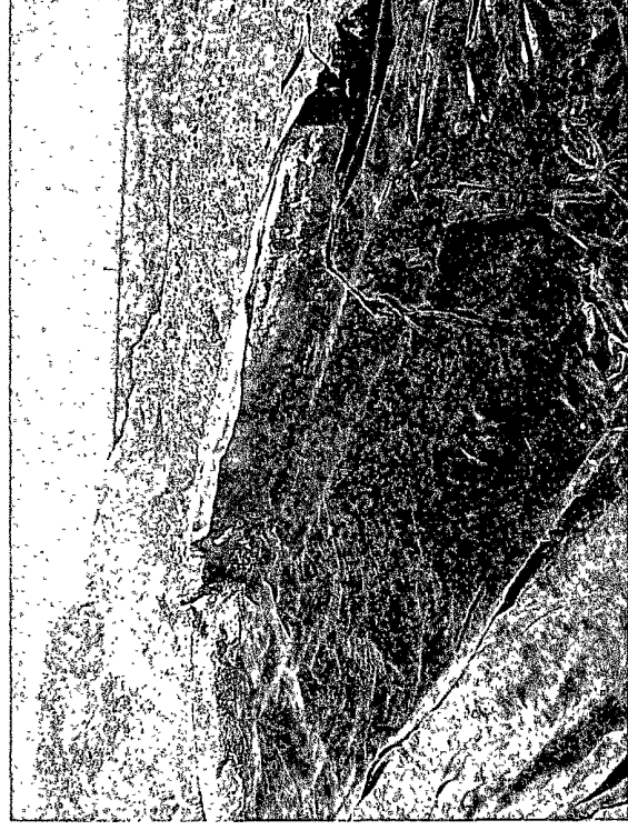
Burial pit #1 capped with a 20 mil poly liner.
