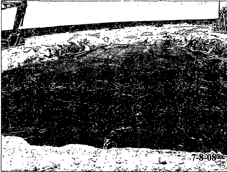
Burial pit #2 capped with a 20 mil poly liner.
