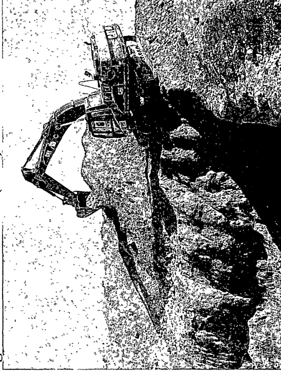
Trackhoe excavating contamination below pit.
