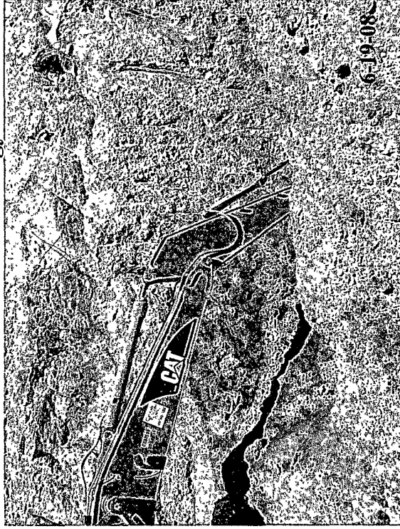
Trackhoe excavating delineation trench below pit.
