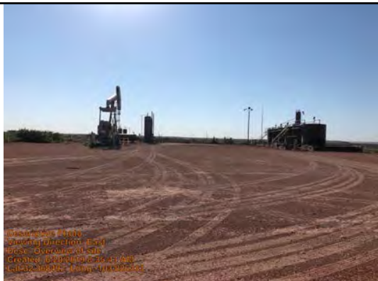
Overview of site
