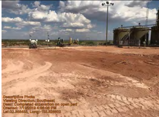
Completed excavation on open pad
