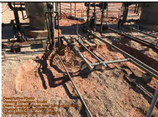
Excavated area near point of release
