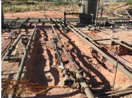
Excavated area within production area
