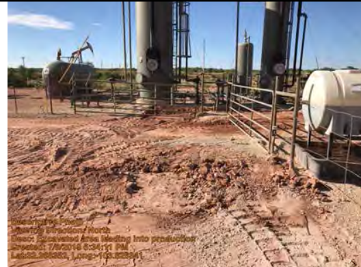
Excavated area leading into production
