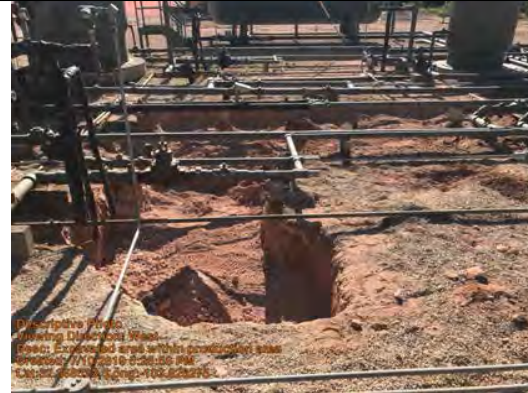
Excavated area within production area
