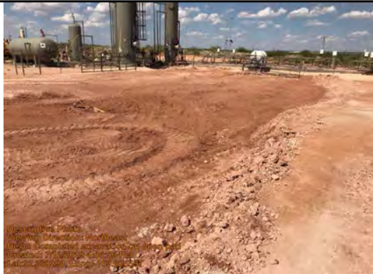
Completed excavation on open pad
