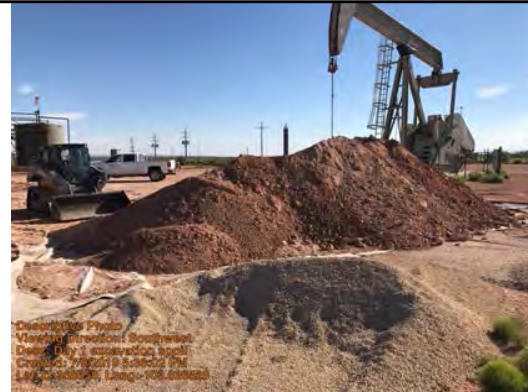
Day 1 excavation spoil
