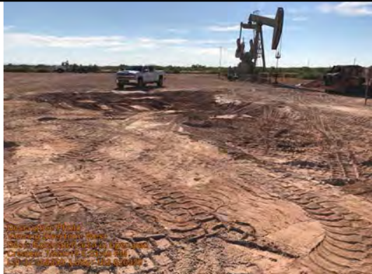
Excavated area in open pad
