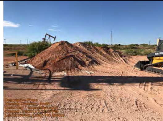
Day 1 excavation spoil
