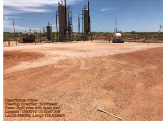
Spill area into open pad
