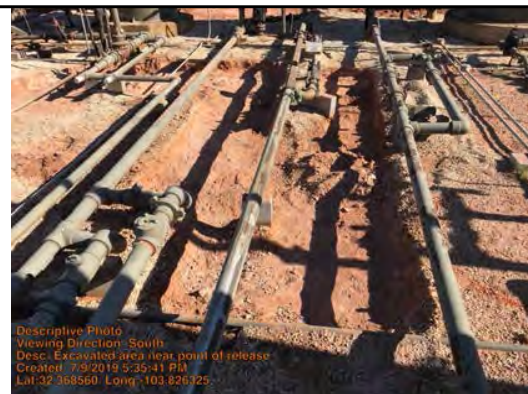
Excavated area near point of release
