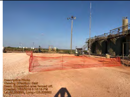
Excavation area fenced off.
