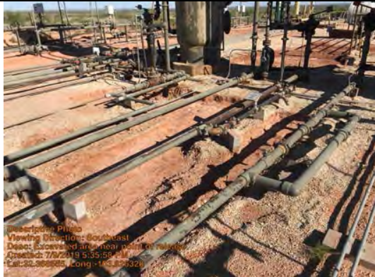
Excavated area near point of release
