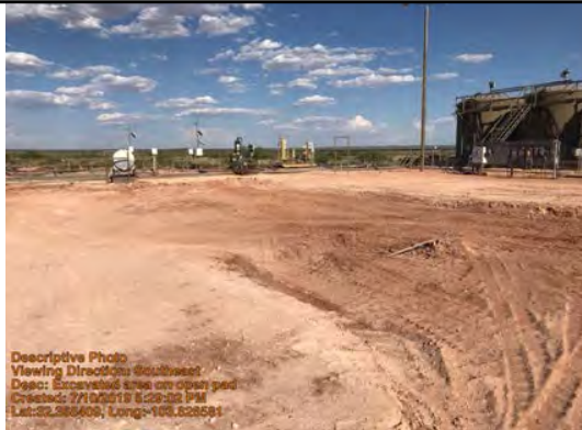
Excavated area on open pad
