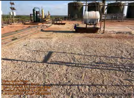
Viewing Direction: South
