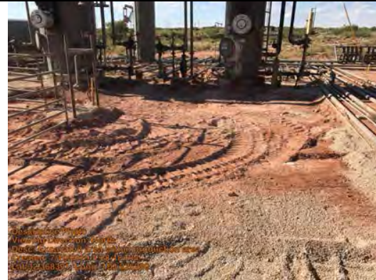
Excavated area within production area
