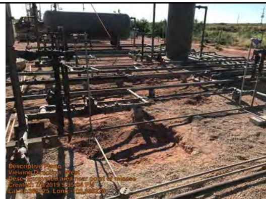
Excavated area near point of release
