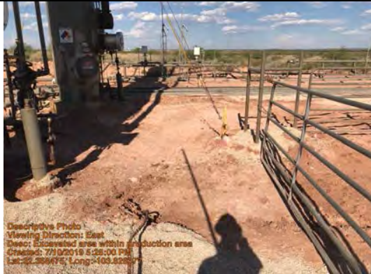
Excavated area within production area
