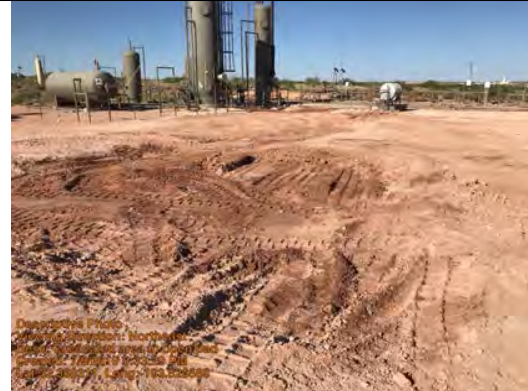
Excavated area in open pad
