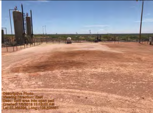
Spill area into open pad
