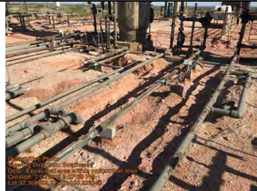
Excavated area within production area
