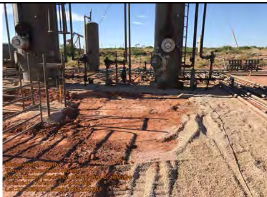
Excavated area near point of release
