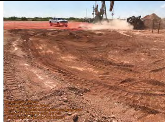
Completed excavation on open pad
