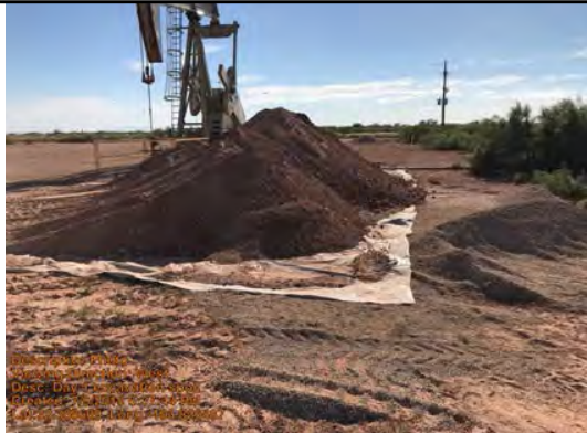
Day 1 excavation spoil
