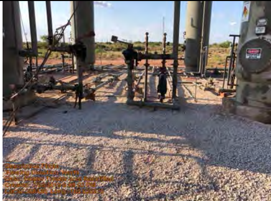
Heater Treater area backfilled.
