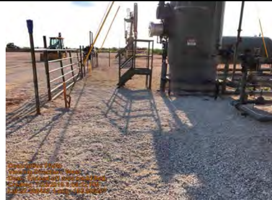
Viewing Direction: West
