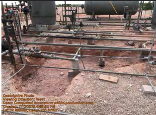
Viewing Direction: West
