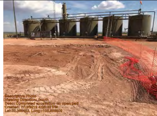
Completed excavation on open pad
