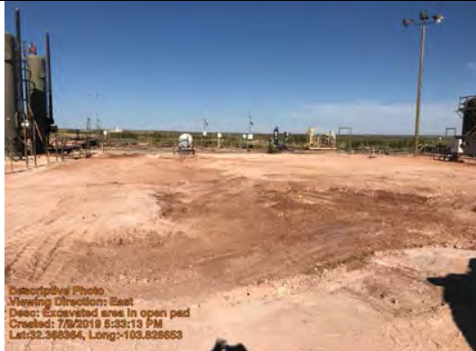
Excavated area in open pad
