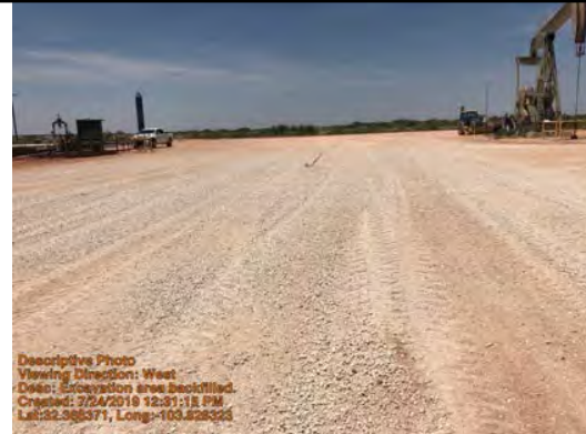
Viewing Direction: West
