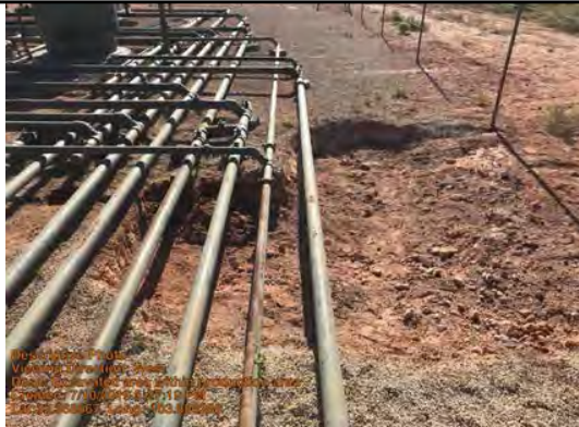
Excavated area within production area
