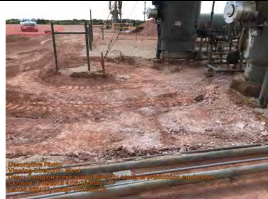
Viewing Direction: West
