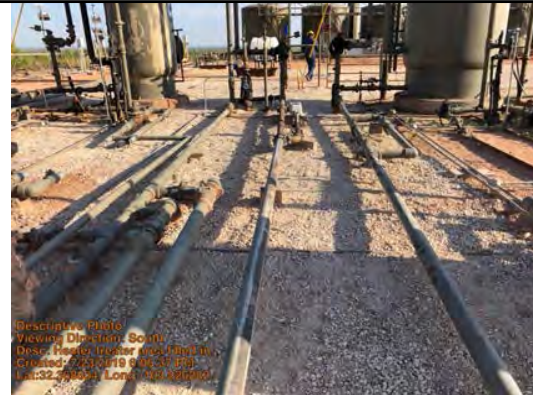
Viewing Direction: South
