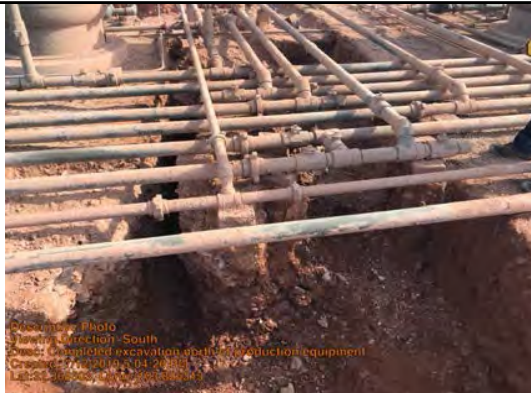
Viewing Direction: South
