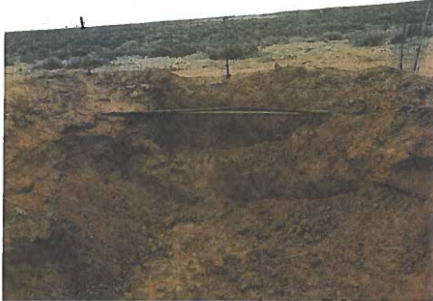
Photo 1: BGT excavation facing northeast. Photo taken December 21, 2018.
