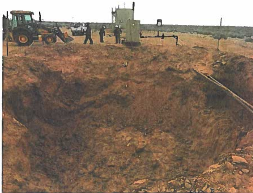
Photo 2: BGT excavation facing northwest towards the separator. Photo taken December 21, 2018.
