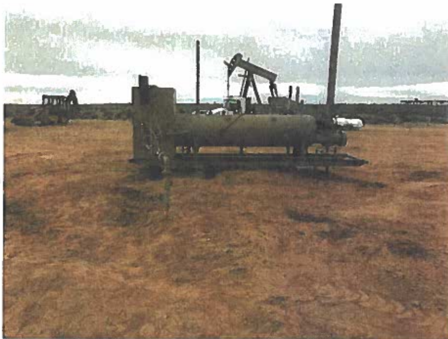
Photo 6: Excavation of surficial soils from separator release. Photo taken December 21, 2018.
