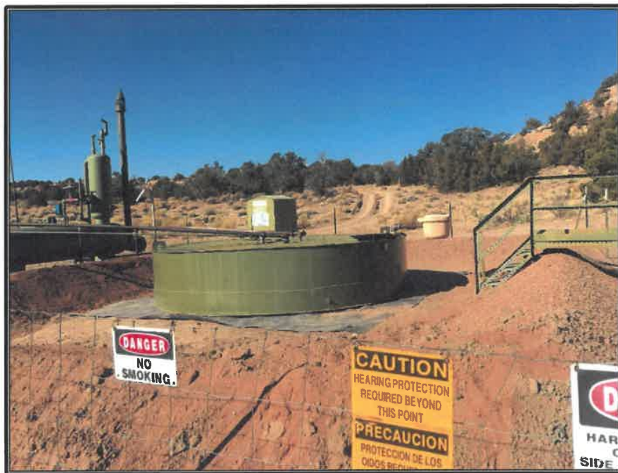
PHOTO 1: Tank Replacing Closed BGT (View 1)
