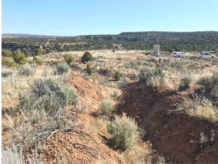
Figure 17. Erosion atop cut slope.
