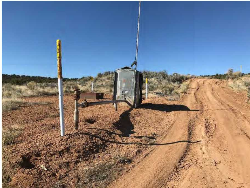
Figure 6. Meter run and above grade pit to remain on the edge of the reclaimed location.
