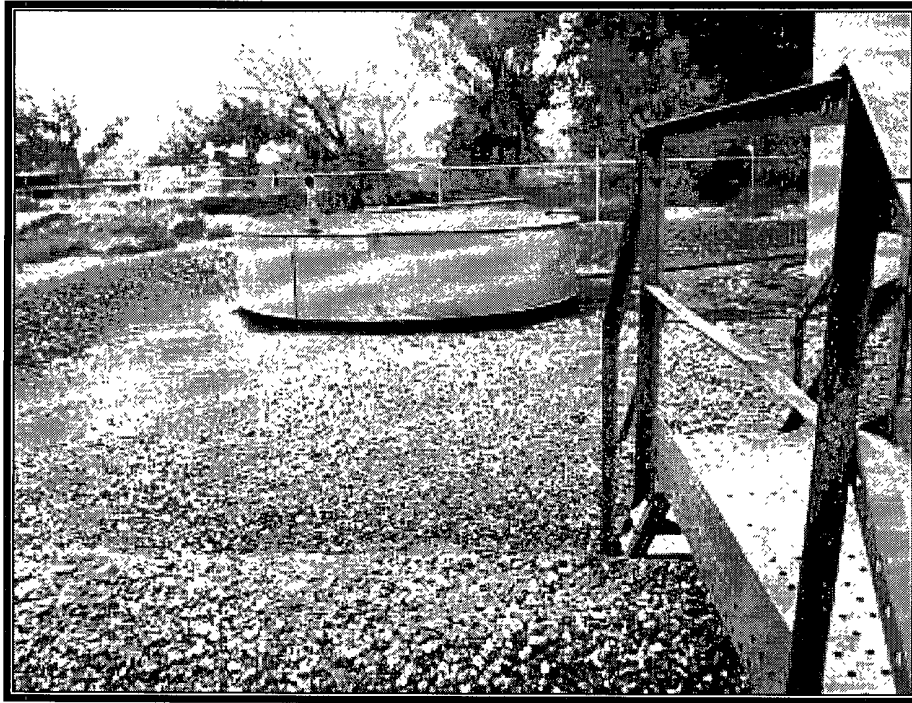
Photo 1: Payne A #1 after Backfill and Tank re-set (View 1)
