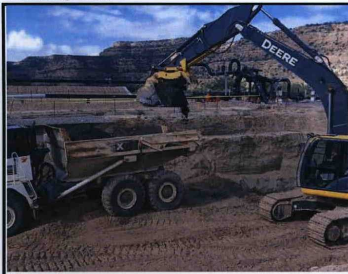
3.) Representative view of the excavation of affected soils from Area 1.
