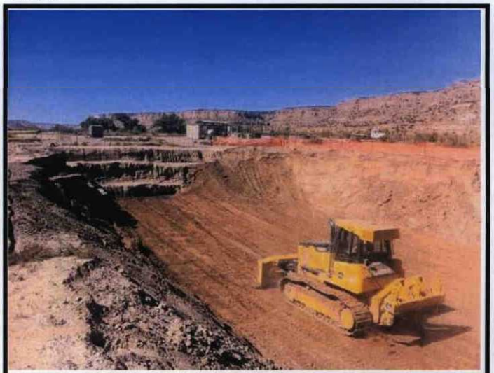
4.) Representative view of the backfilling of Area 1 with unaffected soil.
