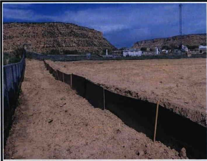
1.) General view of the construction of the treatment cells and surrounding silt fence.
