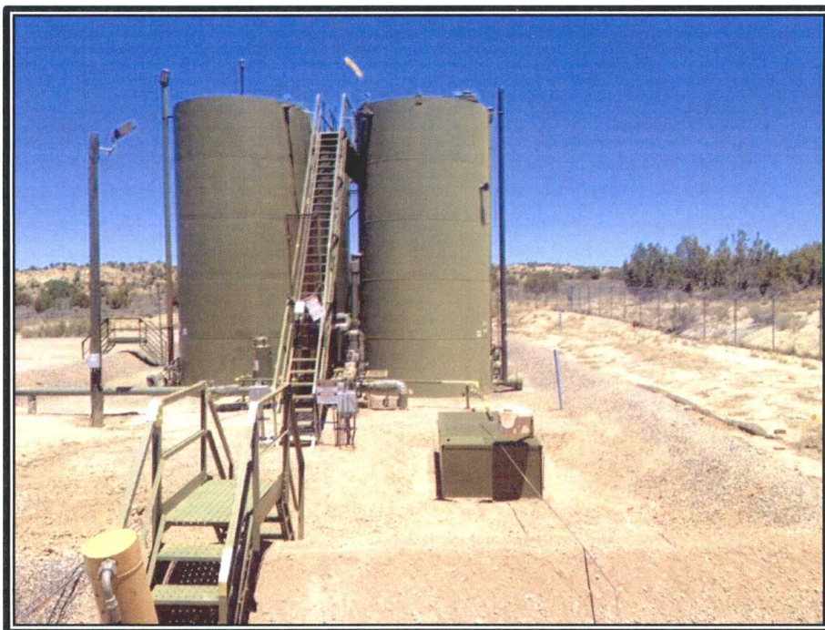
PHOTO 1: BGT Area after set of new Above Grade Tank
