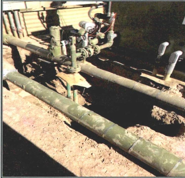
PHOTO 1: Spill Area after excavation
