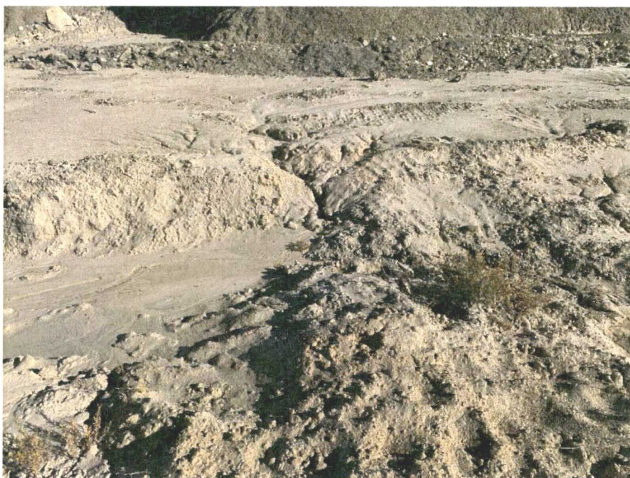
Photo 4: Excavation area along surface drainage.
