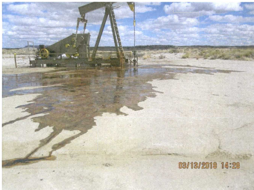
Photo 1: The site before excavation took place.
