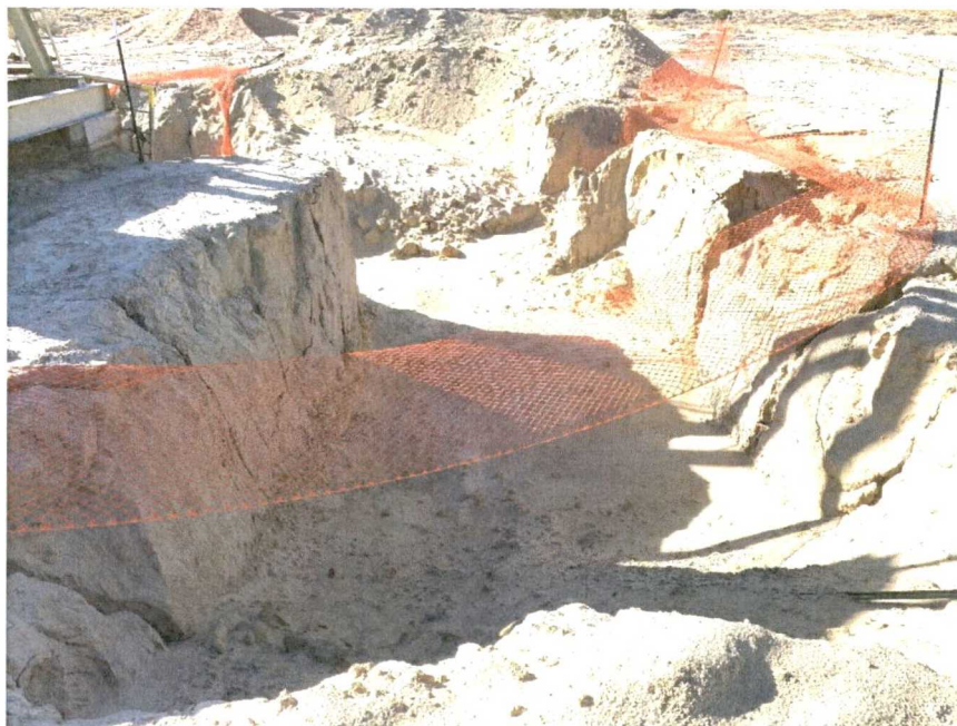
Photo 3: Excavation adjacent to pump jack.
