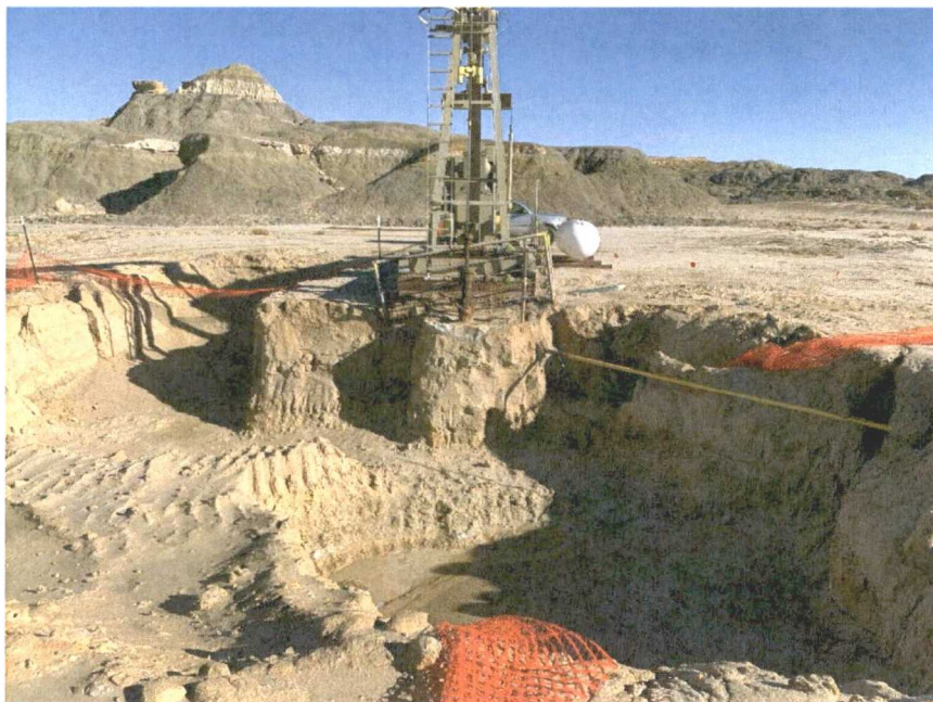
Photo 2: Existing excavation of initial release.
