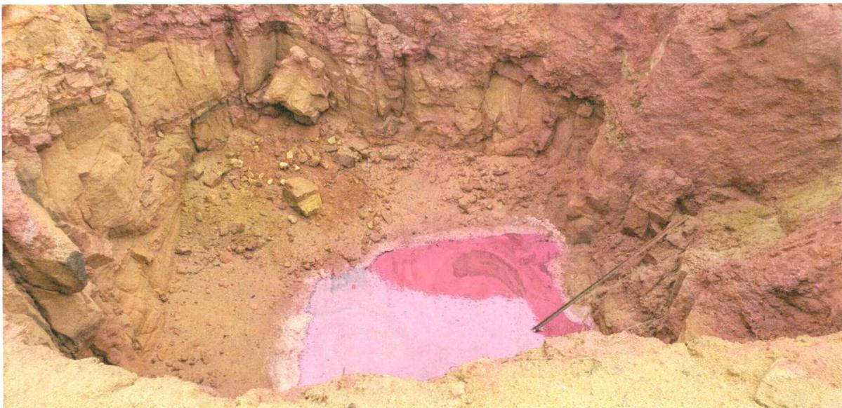
Photo 4: Excavation upon application of potassium permanganate. Photo taken October 24, 2018.
