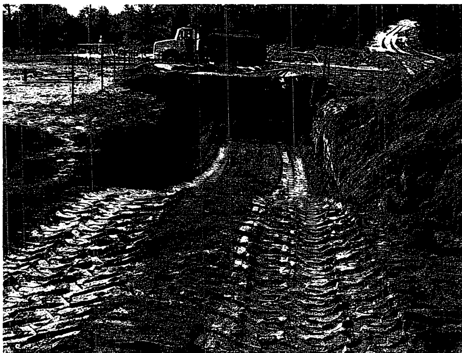
Photo 8: Excavation and contaminated soil on dump truck.
