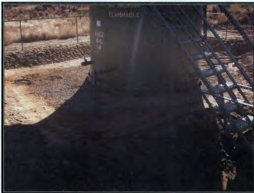
Photo 1: Stained Area Around AST #1
