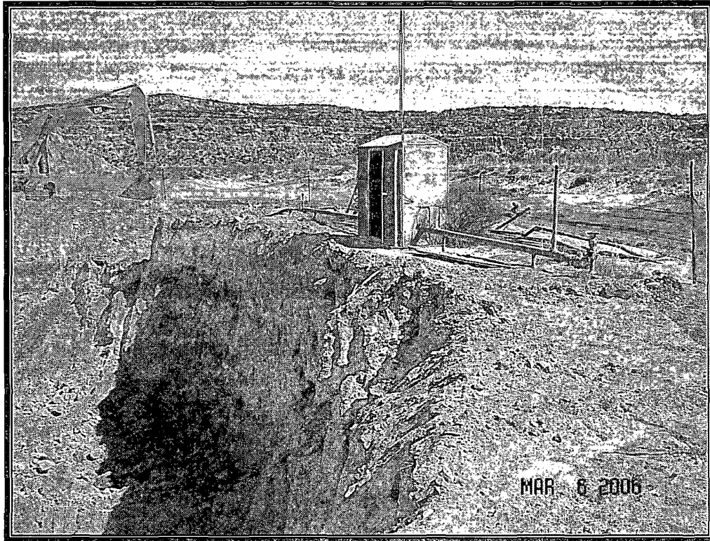
Photo 13: East wall, excavated to below NMOCD guidelines
