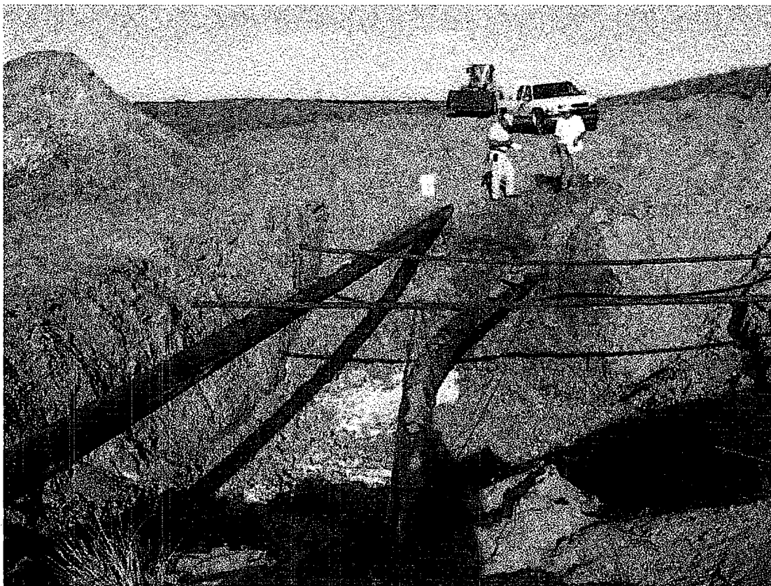
3 View facing west showing hydrocarbon-stained soil on the west wall between the out of service pipeline (left) and in service (right) during excavation activities (06-13-02).
