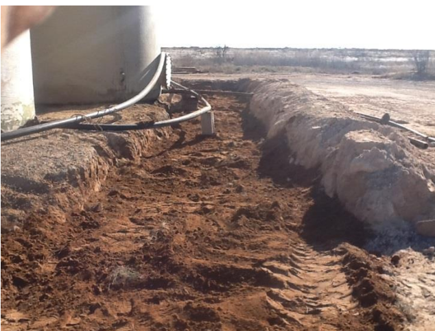
Excavated area west side of tanks
