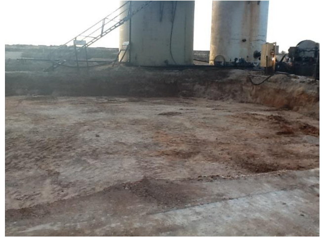
Excavated area facing northwest
