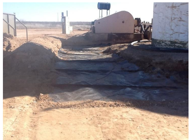
Excavated and lined west side of tanks
