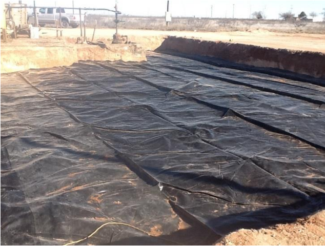
Lined Excavation facing north
