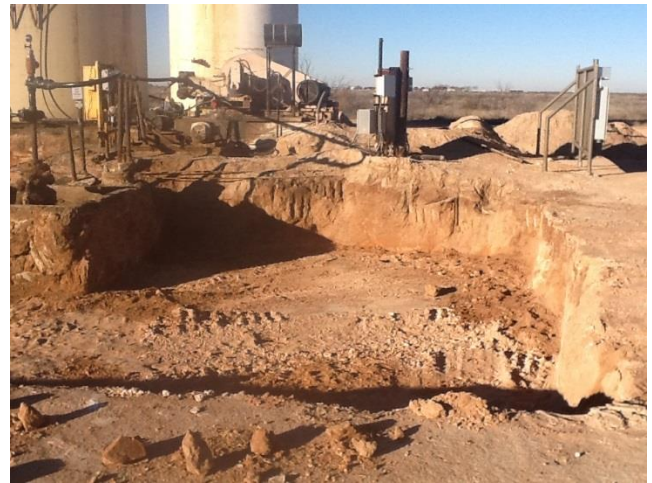
Excavated area northwest
