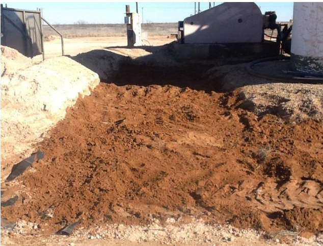
Lined west side of tanks with layered top soil
