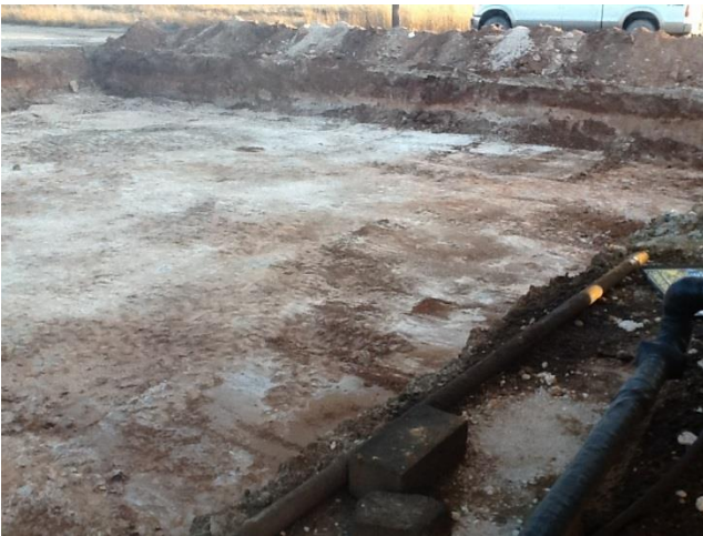
Excavated area South of battery
