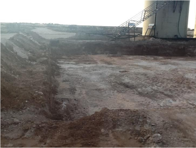
Excavated area facing west
