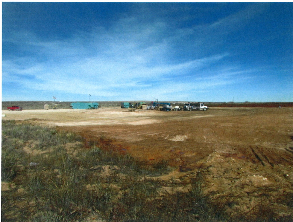
Viewing Northeast from Southwest Corner of Location December 5, 2015
