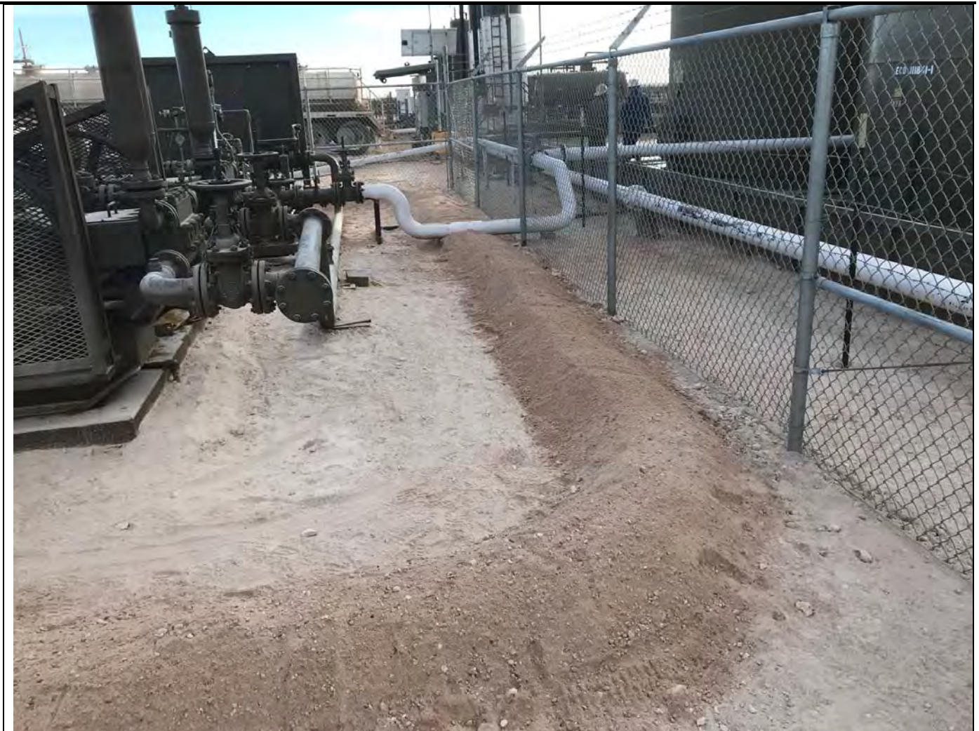
Photo 9: View of the affected area after remediation activities, facing south.
