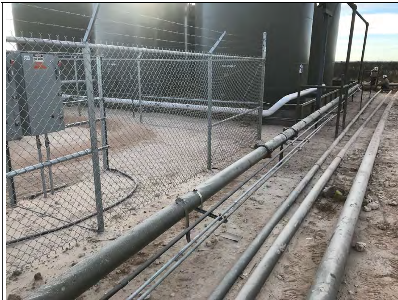
Photo 10: View of the affected area after remediation activities, facing west.
