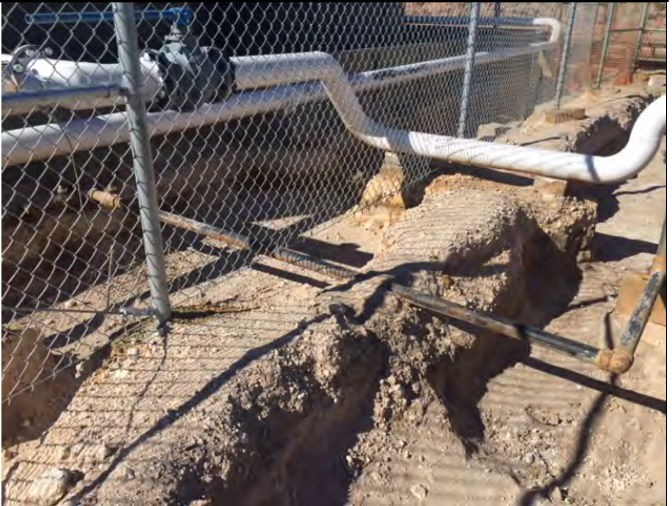
Photo 7: View of portion of the excavated area, facing northwest.
