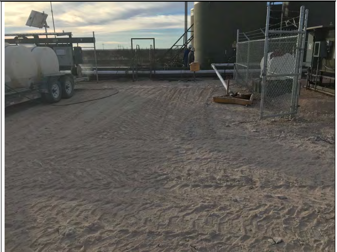
Photo 8: View of the affected area after remediation activities, facing west.
