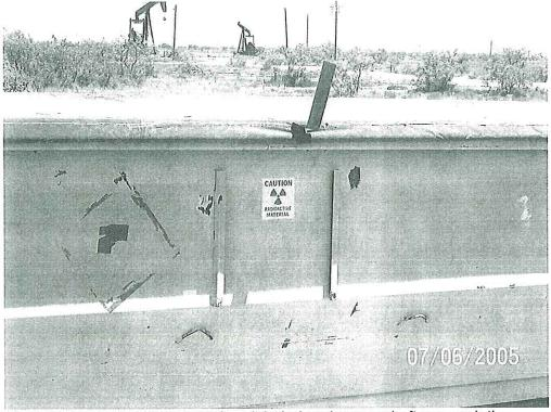
Photo 6: Roll-off NORM container labeled and covered after completion of NORM removal activity.
