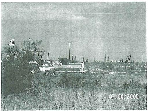
Photo 5: Transfer of NORM-containing material to the roll-off storage container.
