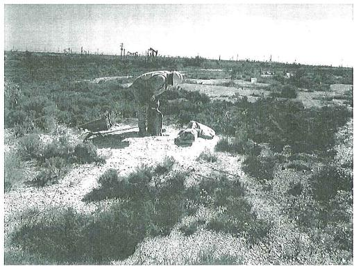
Photo 10: Plugging soil boring with bentonite. Date: August 23, 2005.
