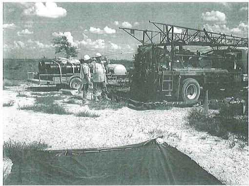
Photo 9: Decontaminating drill rig between boring locations. Date: August 22, 2005.
