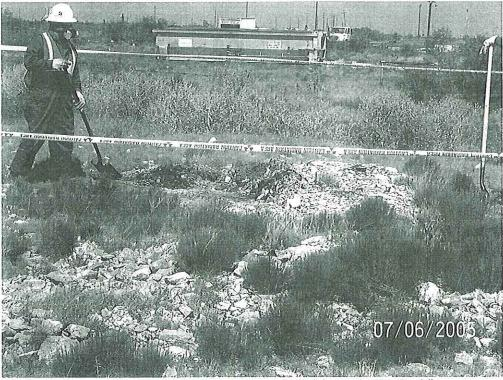
Photo 4: Removal of NORM-containing material from the "1 Grab" sample location.
