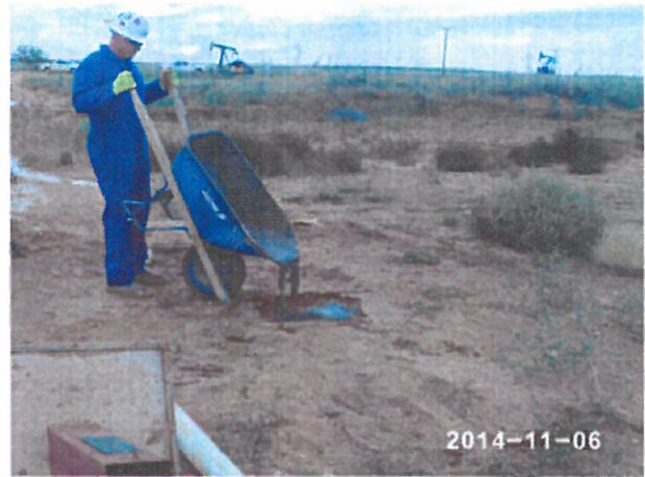
Plugging MW-1R with a Portland/Bentonite slurry and a 3 ft concrete cap, facing west 11/6/2014
