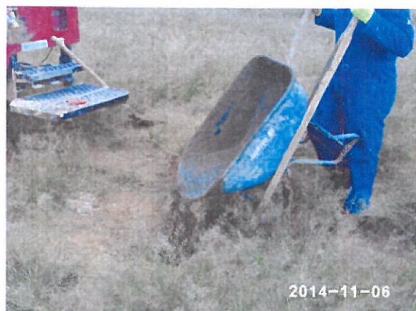
Plugging MW-5 with a Portland/Bentonite slurry and a 3 ft concrete cap, facing north 11/6/2014
