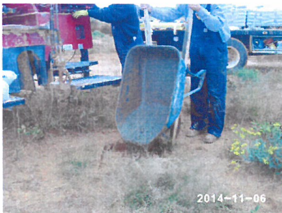
Plugging MW-2 with a Portland/Bentonite slurry and a 3 ft concrete cap, facing north 11/6/2014
