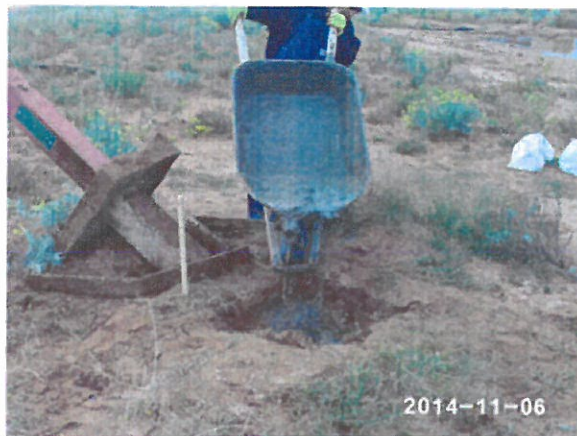
Plugging MW-3 with a Portland/Bentonite slurry and a 3 ft concrete cap, facing south 11/6/2014
