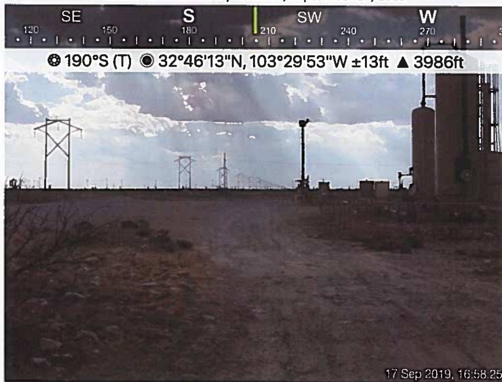
Site Viewing Southwest, September 17, 2019
