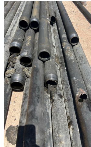
Figure 8. Corroded Production Tubing
