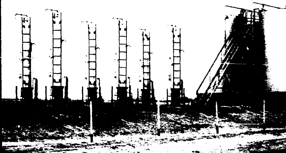
A central battery of six National Two-Phase Metering Separators in Southern Oklahoma, producing three wells, two zones each, commingling, into one tank battery. (Shown top.)
