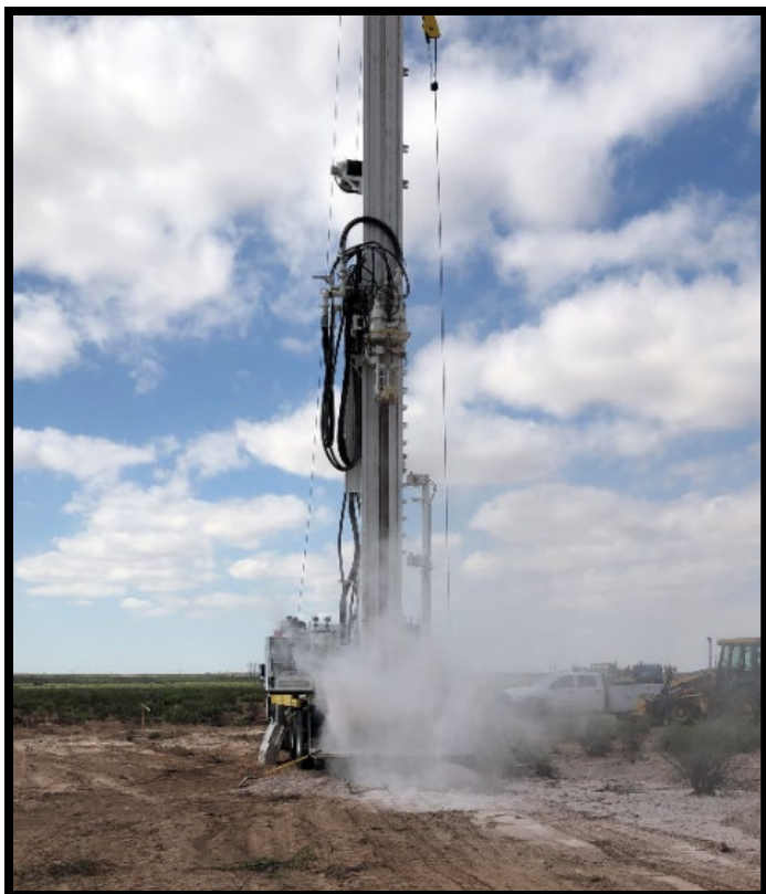
Image 1 - Drilling through dry gypsiferous soils.
