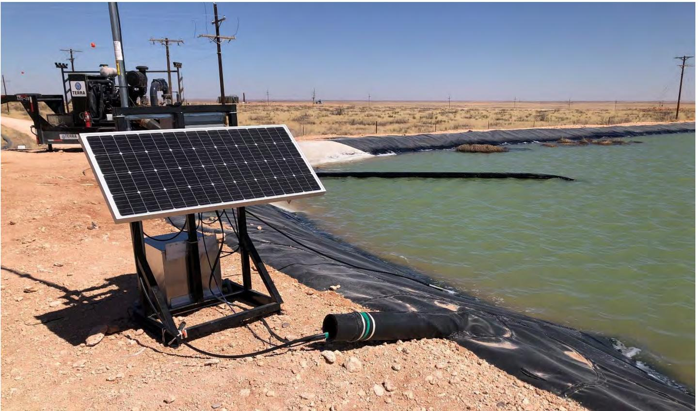
SP-1A Northwest corner of Gamma Ridge Containment #1 showing leak detection system
