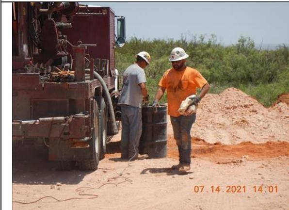
Photo 3 Grouting Borehole #2.
