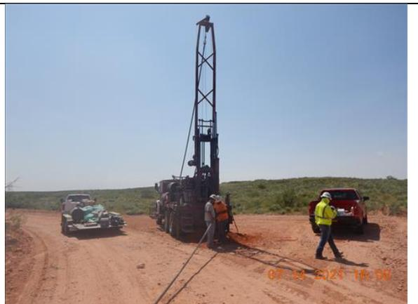
Photo 6 Drilling Borehole #1.
