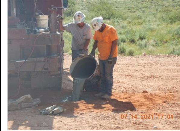
Photo 7 Grouting Borehole #1.
