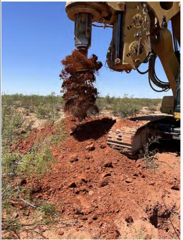
Due to the lack of groundwater data in the area, Solaris elected to drill an auger boring to 75 feet. This auger spin from total depth (74.33 feet) testifies to the dry boring.
