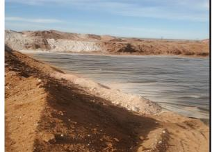
Photo 3: Overview of liner installation.
