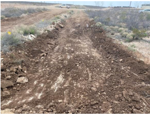
Photograph 9: View of southern excavation in the right of way facing East.
