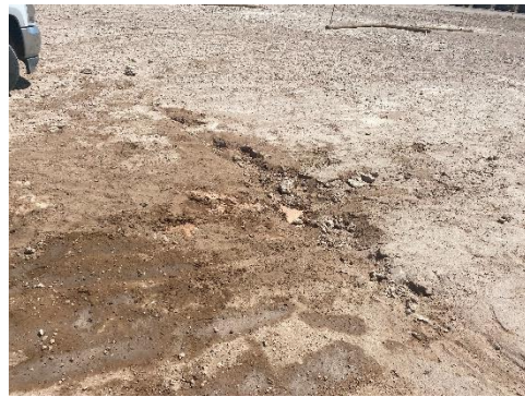
Photograph 22: View of the backfilled core hole area associated with CH07.
