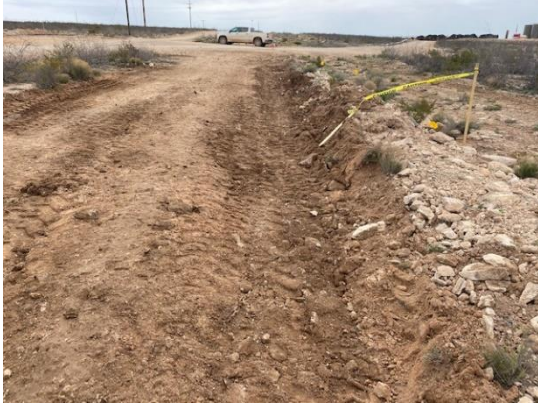
Photograph 7: View of northern excavation in the right of way facing East.
