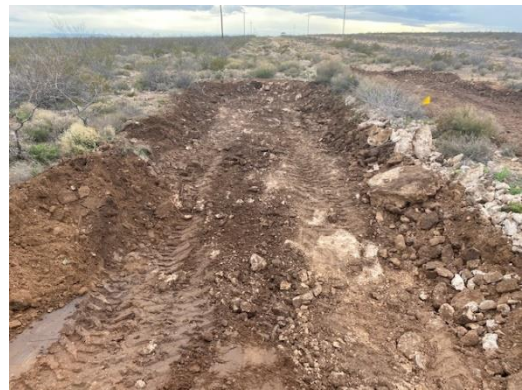
Photograph 10: View of southern excavation in the right of way facing West.
