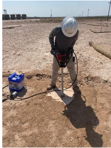
Photograph 20: Utilizing the core drill in the CH07 sample location.
