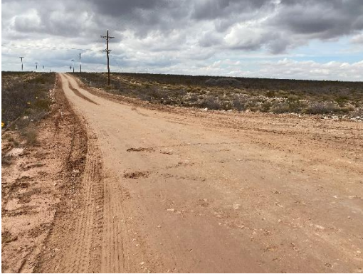
Photograph 1: View of release along lease road.
