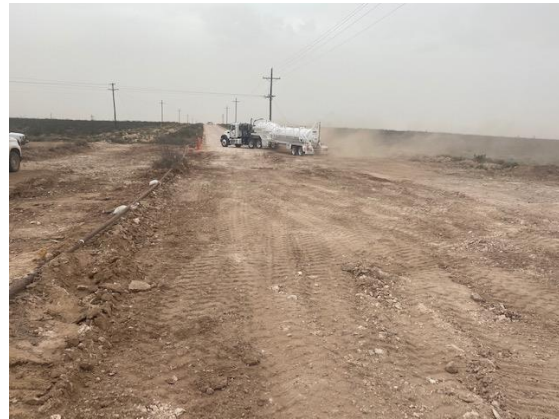
Photograph 14: View of excavation along lease road.
