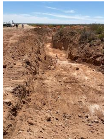
Photograph 16: View of excavation in dry wash.
