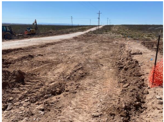
Photograph 12: View of excavation north of lease road facing west.
