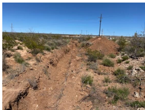
Photograph 18: View of excavation in dry wash facing North.
