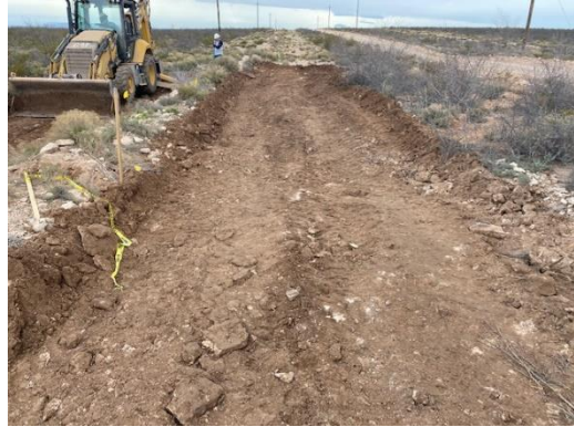
Photograph 8: View of northern excavation in right of way facing West.
