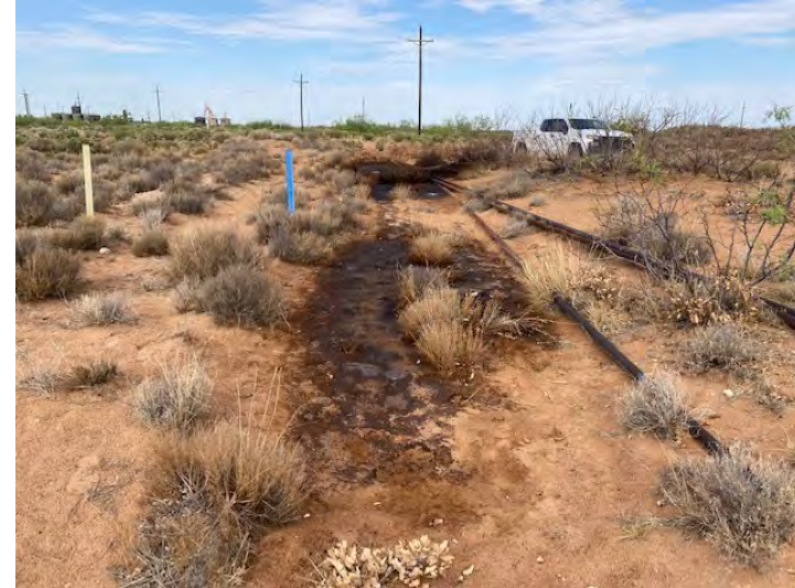
Photograph 2: View of release along steel flowline facing southwest.
