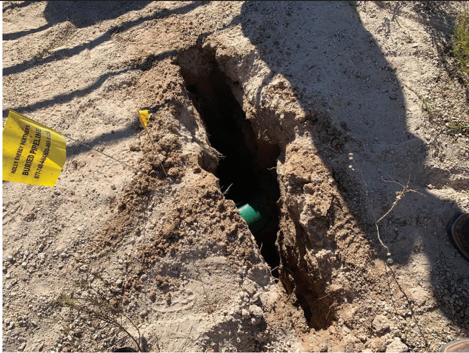
Photo 5: View of the exposed gathering line.
