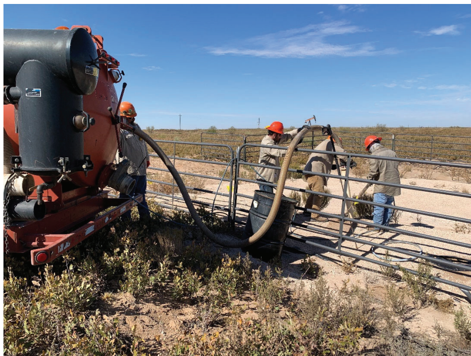
Photo 4: View facing northwest of field crew hydro-excavating across marked location of gathering line to confirm its location and depth.
