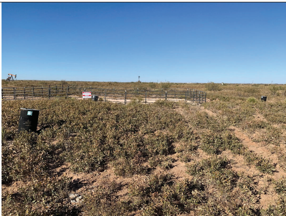
Photo 1: View facing north of fenced former excavation around release point and GHD drums. The drums appear to be associated (from left to right) with SB-2 (left foreground), SB-1 (center background, next to fence), and SB-3 (right background).
