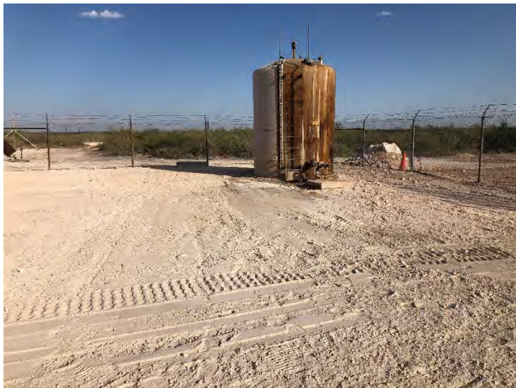
Photograph 9: View of backfill on pad facing East.
