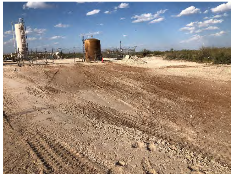
Photograph 10: View of backfill on lease road facing North.
