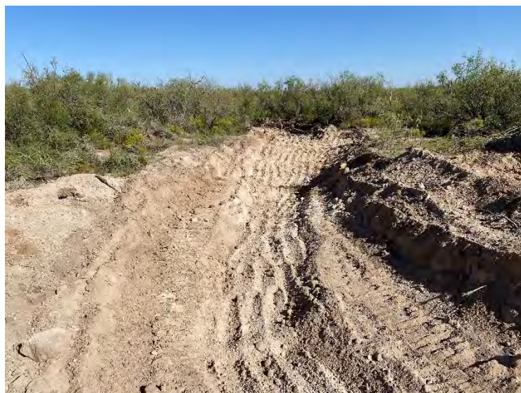
Photograph 7: View of excavation in pasture facing East.
