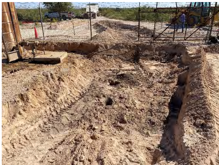
Photograph 5: View of completed excavation on pad facing South.
