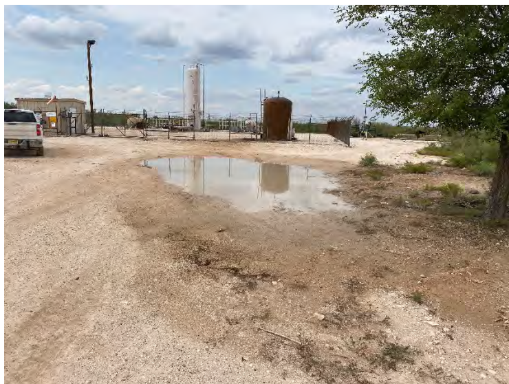
Photograph 1: View of release extent, lease road, and pad facing North.
