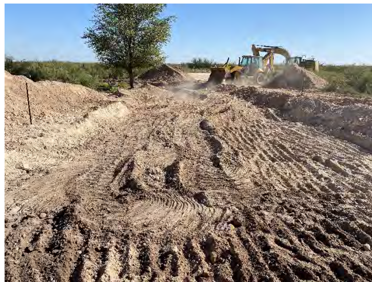
Photograph 6: View of excavation in lease road facing South.
