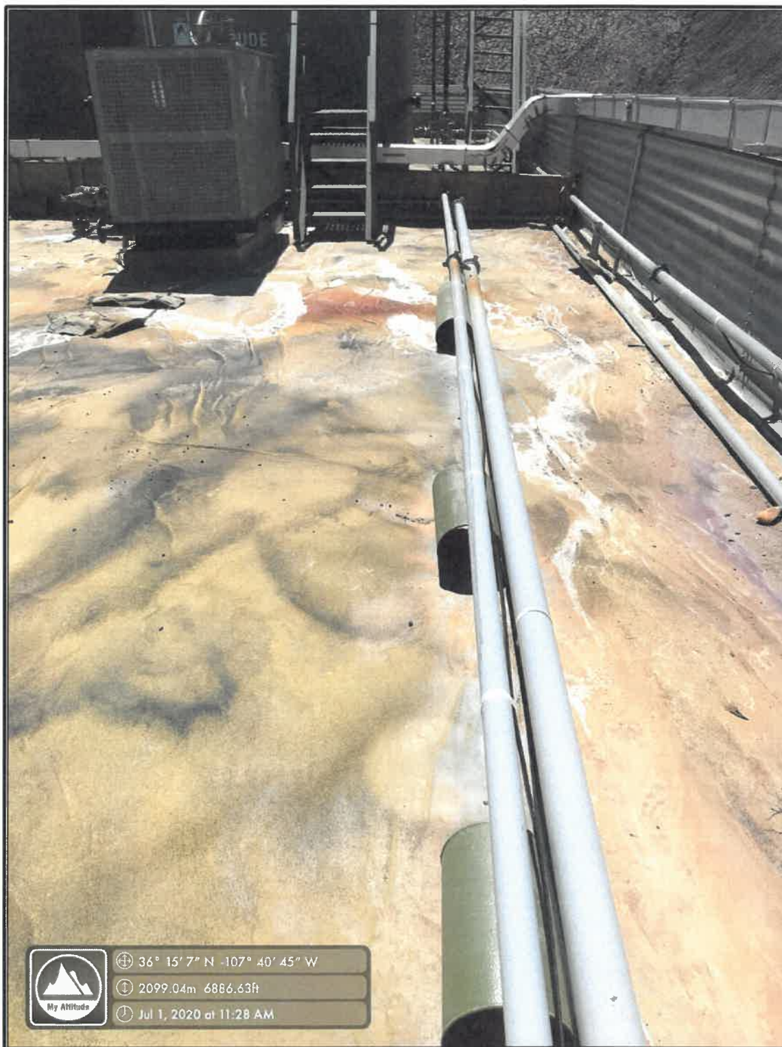
Photo 3: View of Liner after Cleanup
