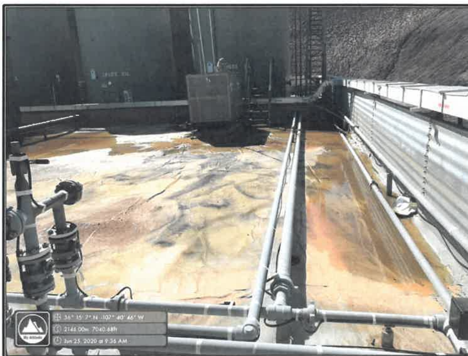
Photo 2: View of Water on Liner
