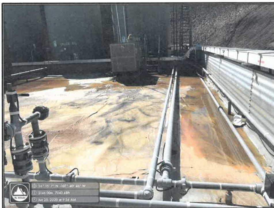
Photo 2: View of Water on Liner
