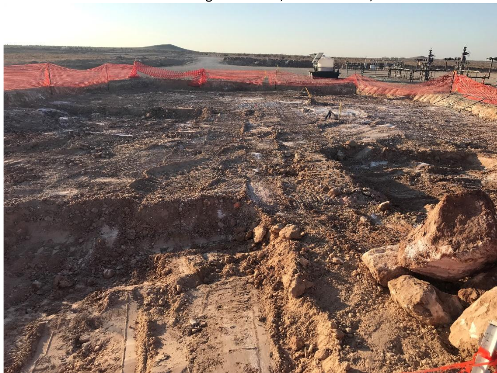
Additional Soil Removed from The Sidewalls (N-SW and S-SW) and Bottom (C'-3, C'-6, C'-14, and C'-20) From The Oil Based Mud Spill Excavation viewing South, November 20, 2020
