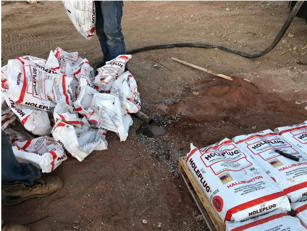
Photo 4: View facing northeast of SB-3 after it was plugged.
