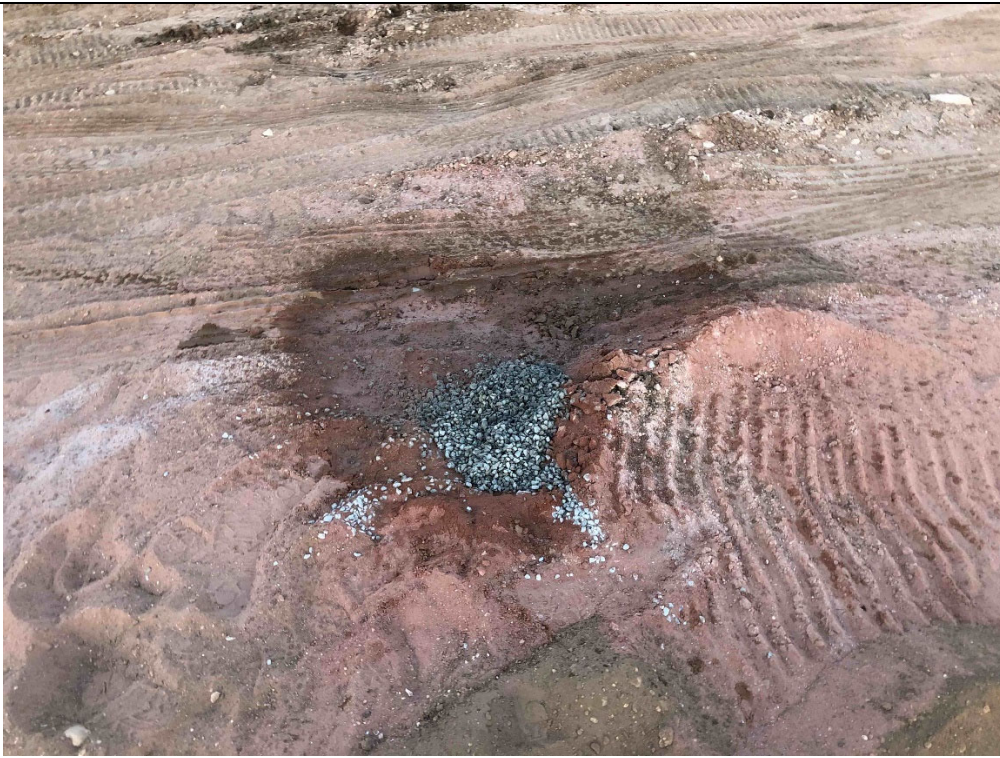
Photo 3: View facing northeast of SB-2 after it was plugged.
