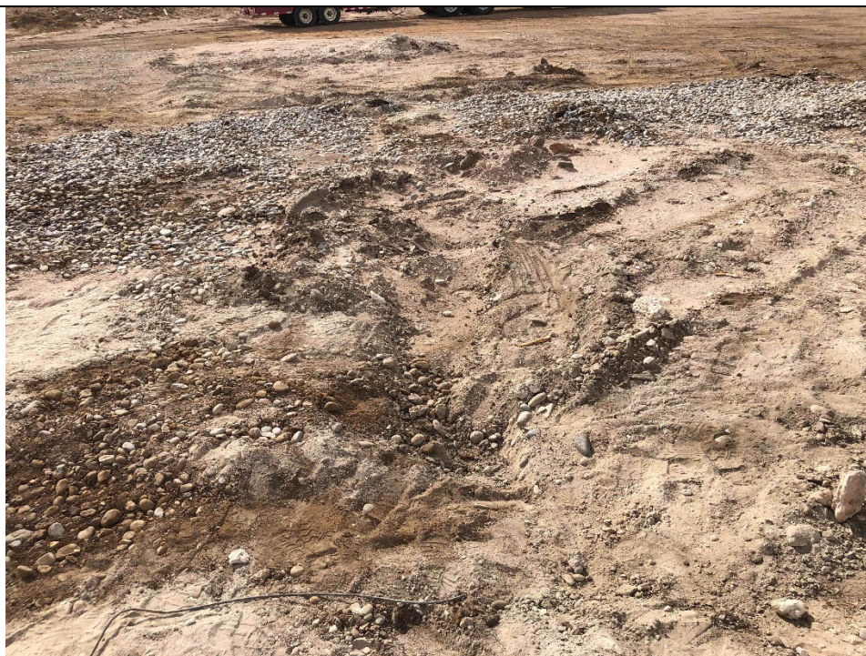
Photo 1: View looking south-southwest of backfilled Test Pit TP-3. Test Pit TP-3 is inside the former Tank 970 footprint and is adjacent to the location of SB-1.
