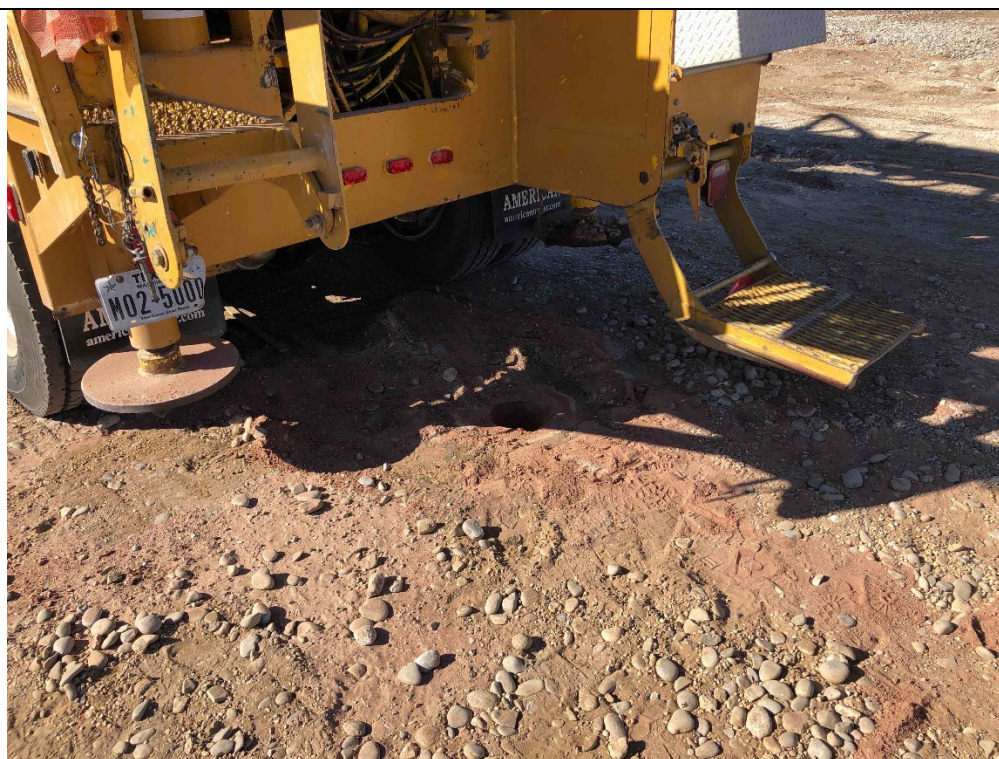
Photo 5: View facing west of SB-4 after installation was complete.
