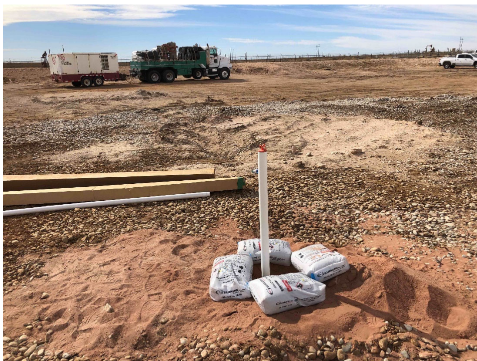
Photo 2: View looking southwest of SB-1. A well casing was installed in SB-1 to prevent the boring from collapsing while standing open for approximately 48 hours to confirm that groundwater was not present at the Site within 100 feet of the ground surface.
