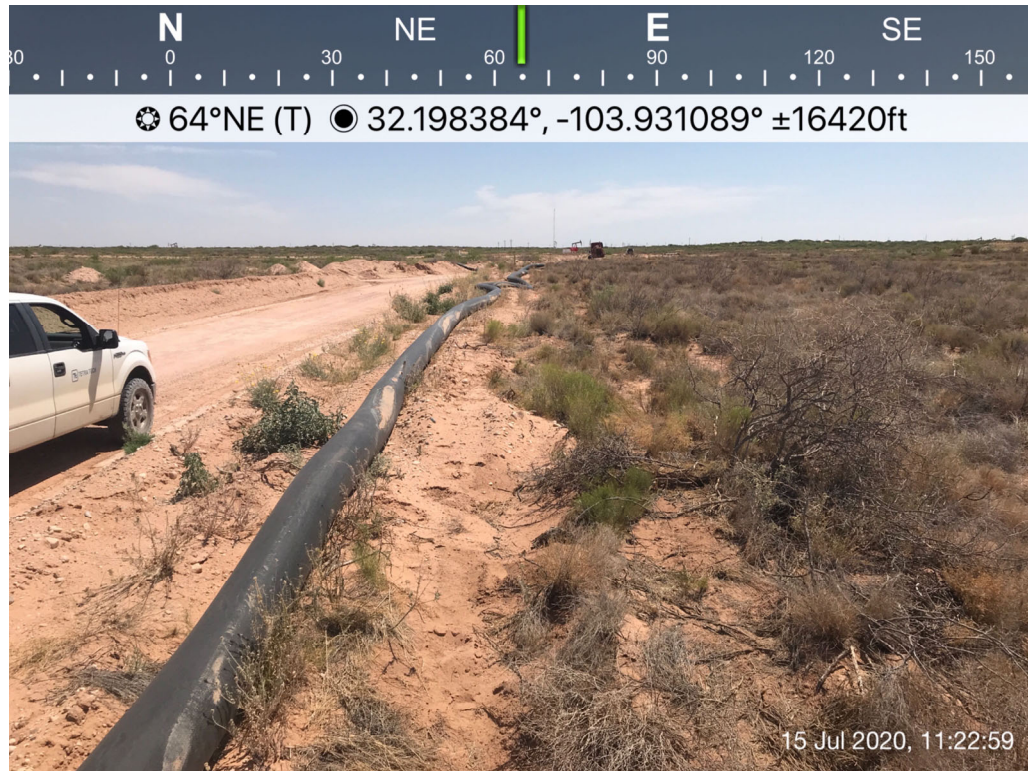
View of Release Area – View Northeast
