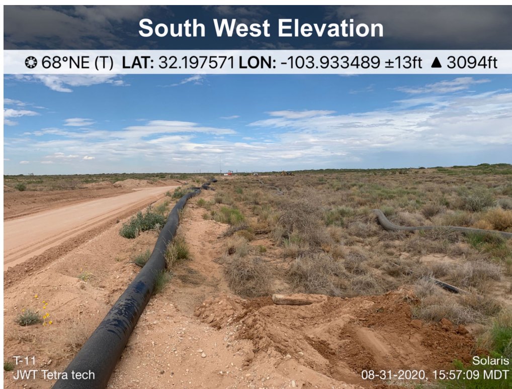
View of Release Area – View Southwest
