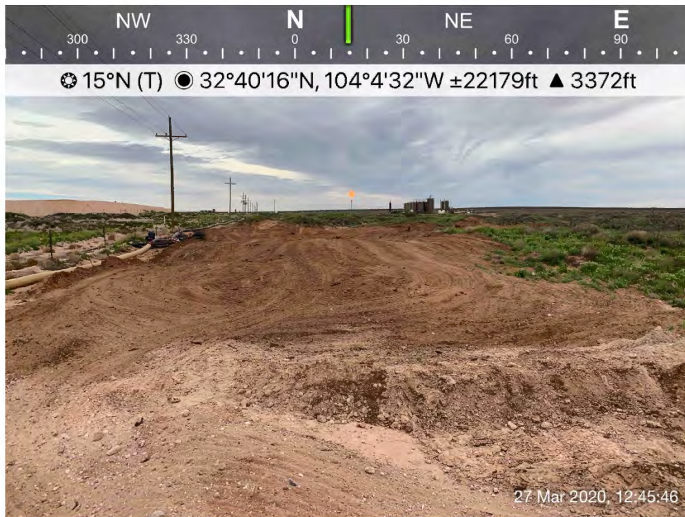
Backfilled and seeded area viewing north
