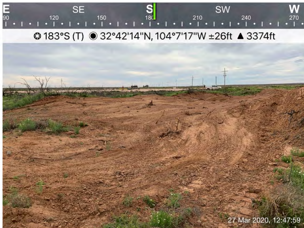
Backfilled and seeded area viewing south
