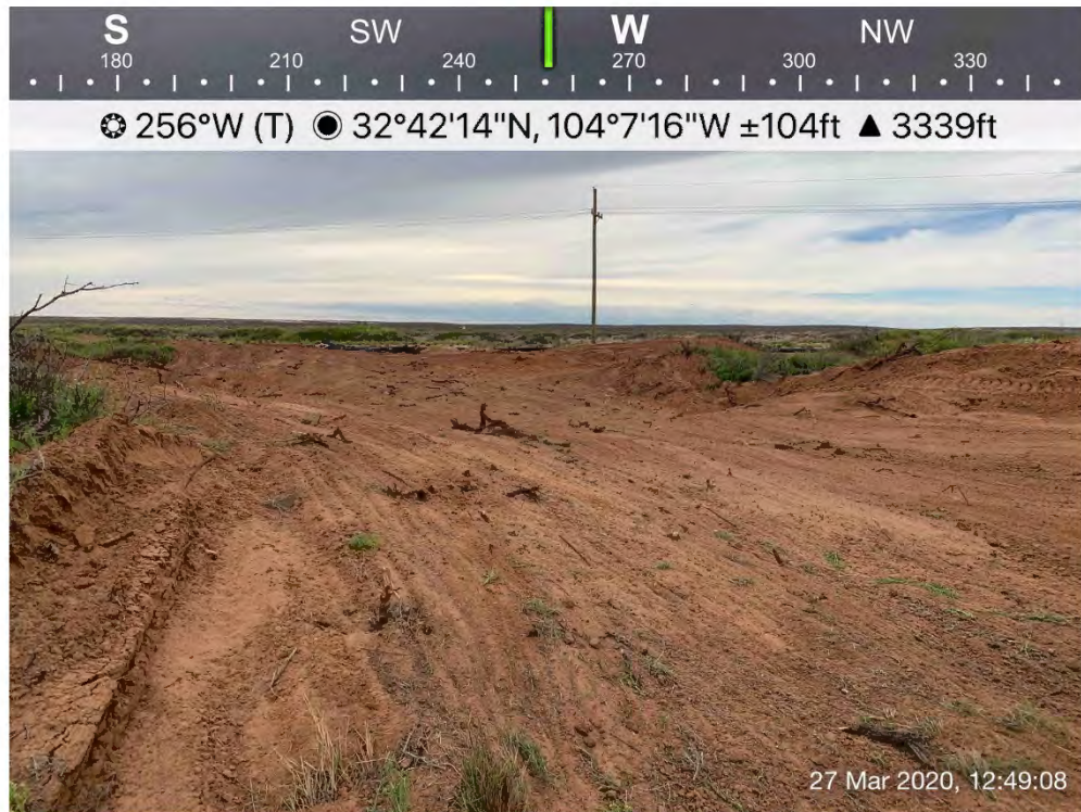
Backfilled and seeded area viewing west
