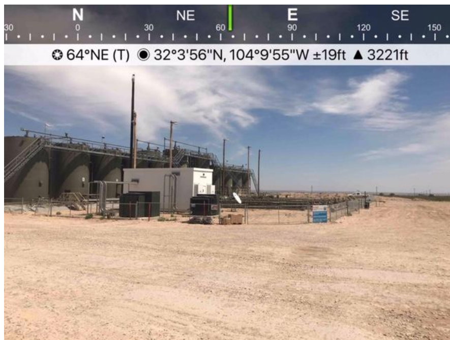
Spill area viewing northeast/east
