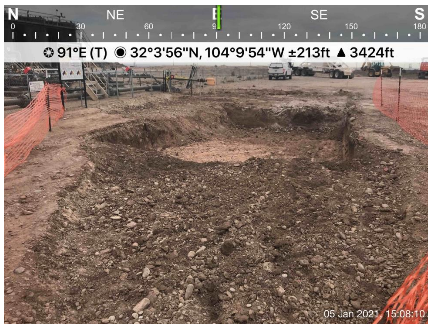
Initially excavated area viewing east, January 5, 2021
