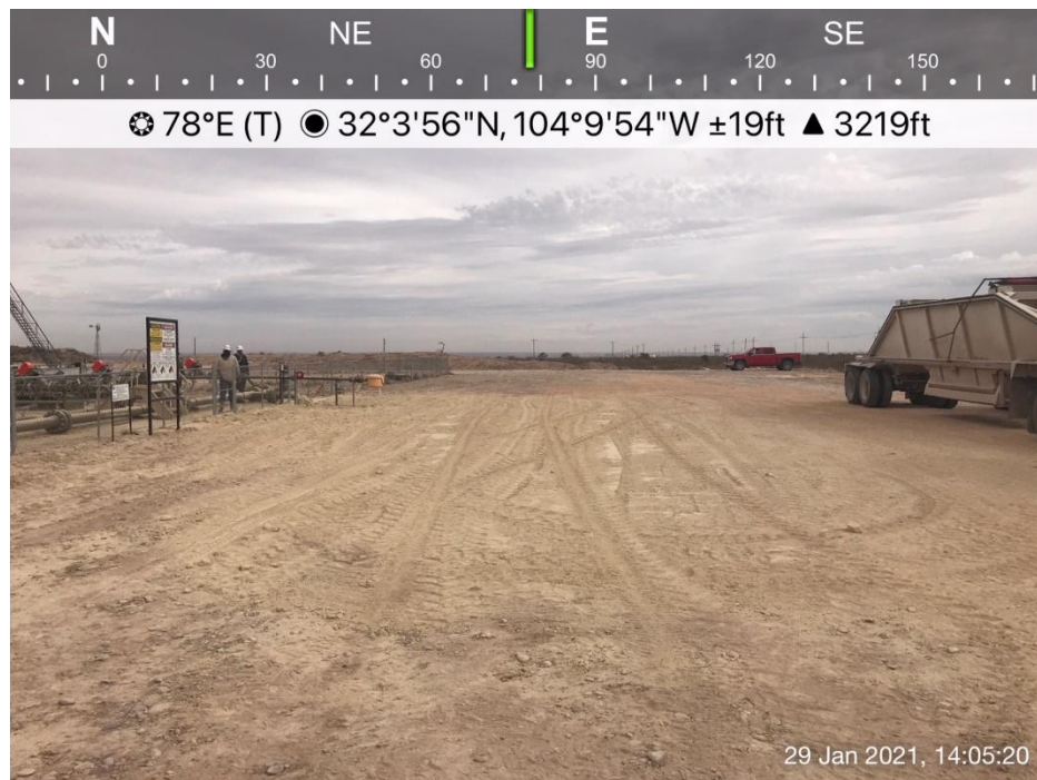
Backfilled excavation, January 29, 2021
