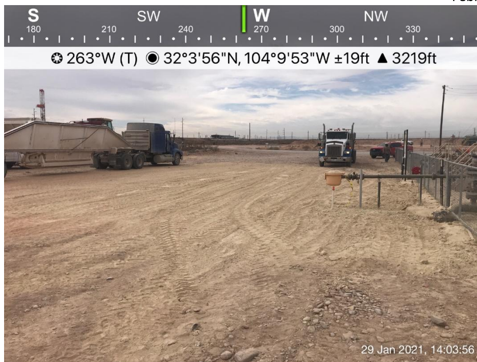
Backfilled excavation, January 29, 2021
