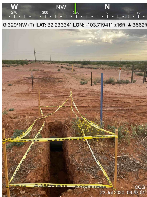
View Northwest – Area of release.
