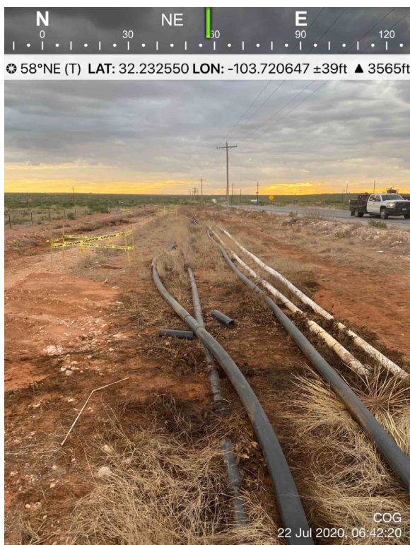
View Northeast – Area of release.
