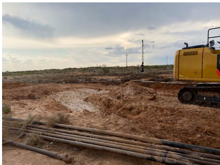
Photograph 7: Northwestern view of excavation towards pasture.
