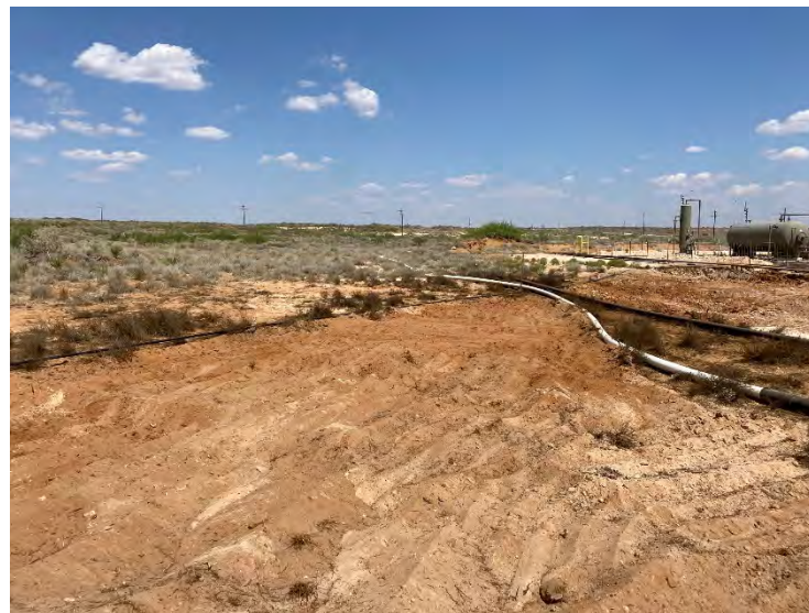
Photograph 10: Backfill in equipment area.
