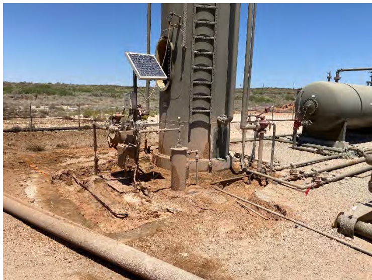
Photograph 5: Northeastern view of hydrovac excavation near equipment.
