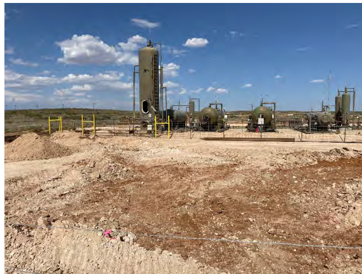
Photograph 6: Eastern view of excavation on pad.
