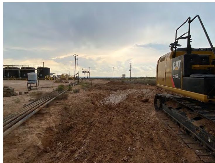
Photograph 8: Western view of excavation.
