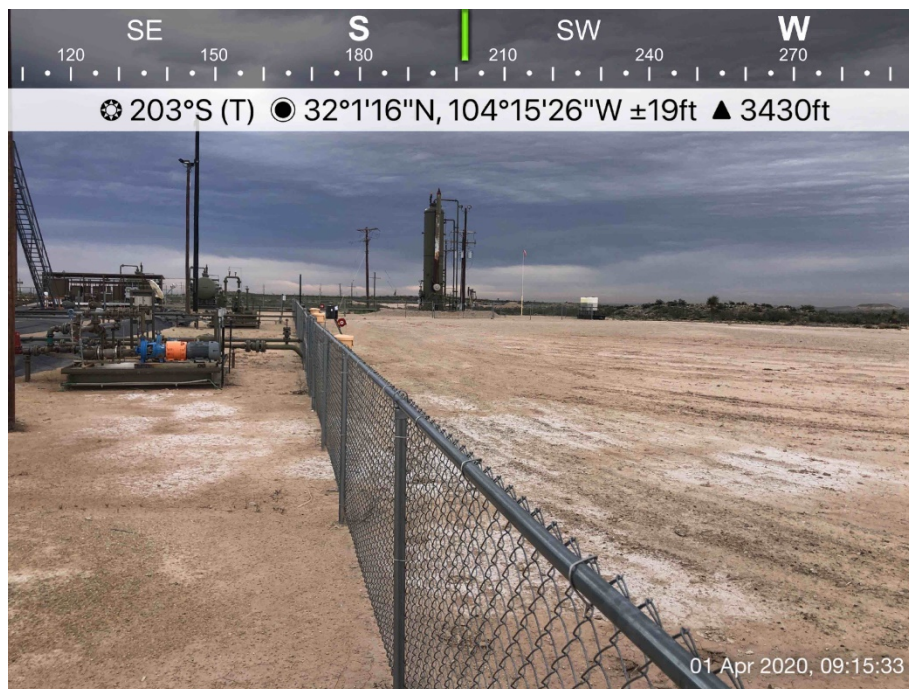
Impacted area viewing south/southwest, April 1, 2020
