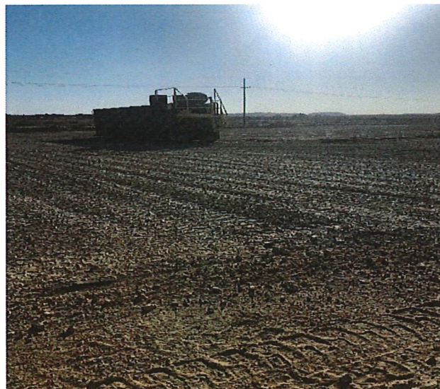
Excavation backfilled to grade
