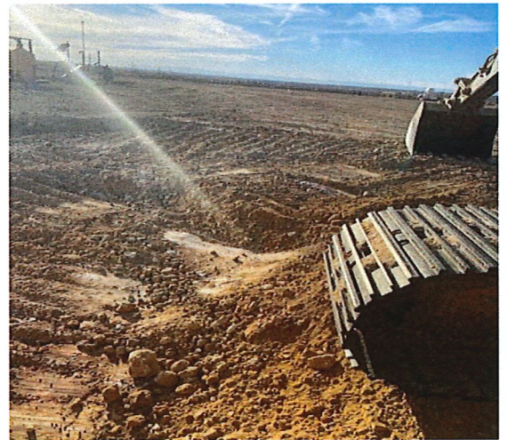
Excavation of Spill Run
