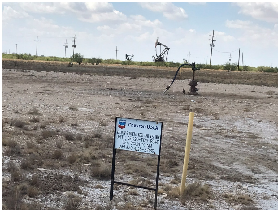
View of location sign and impacted area, September 2, 2020
