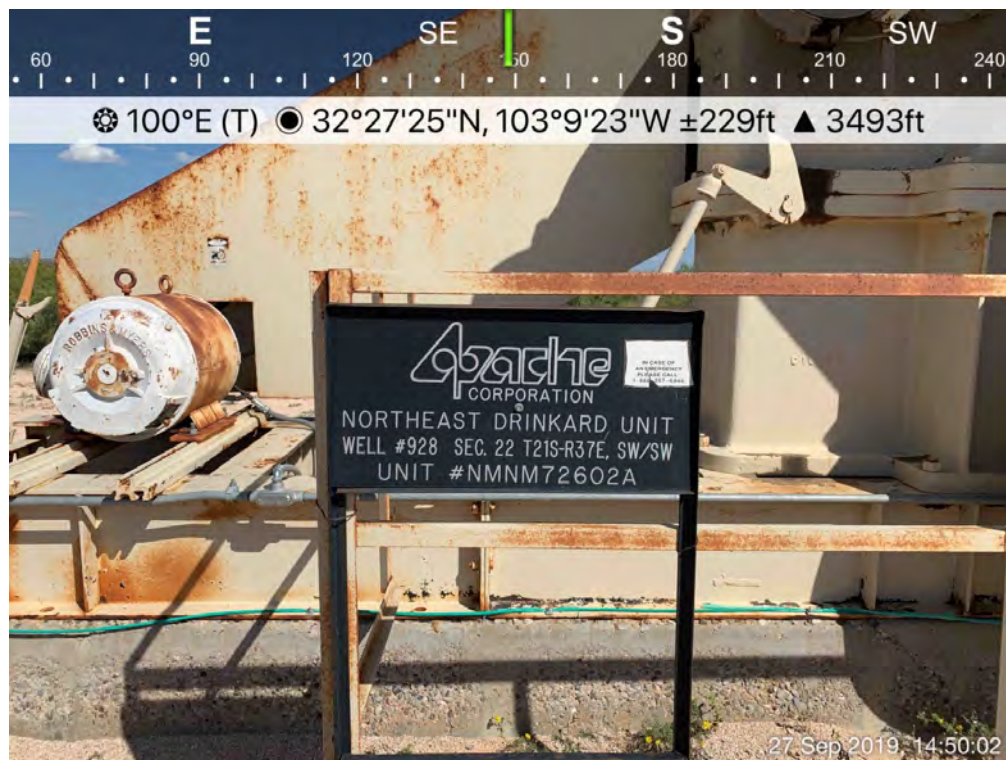
NEDU Well #928 Sign
